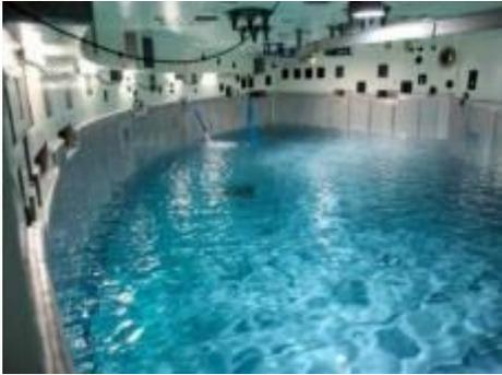
\*In-containment Refueling Water Storage Tank
