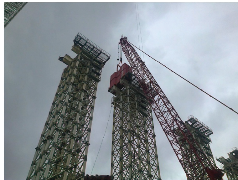
Lifting of Jacking units Set up to the Jacking Tower 3/3
