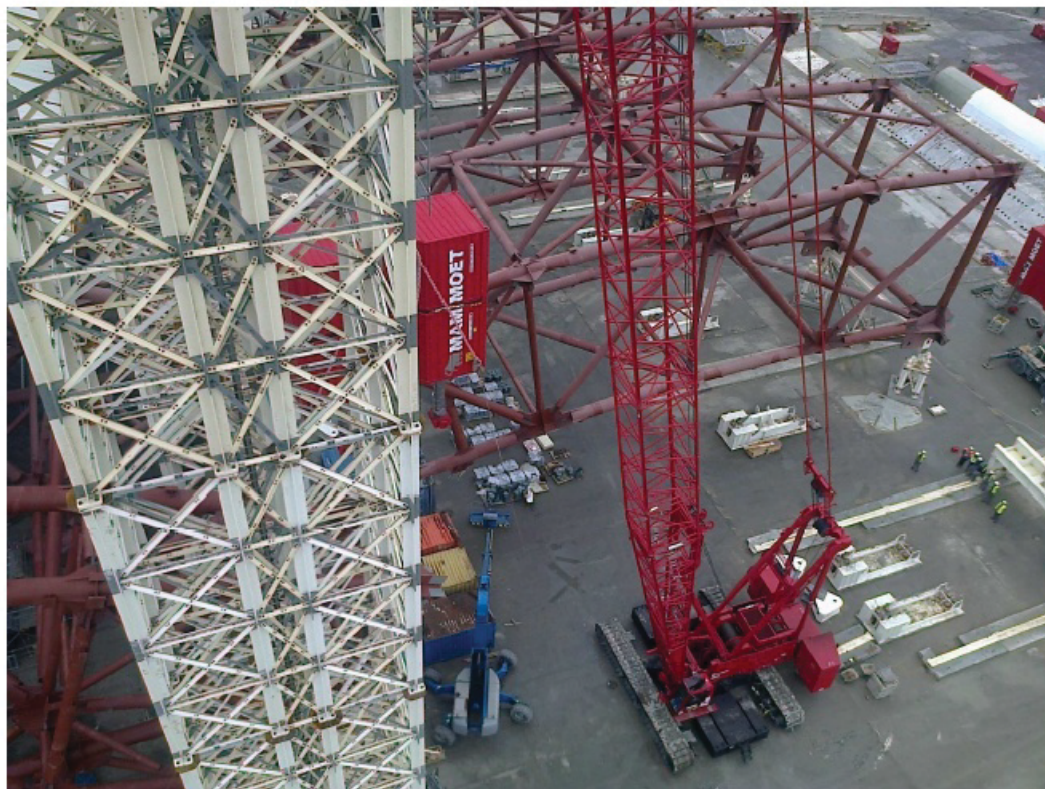
Lifting of Jacking units Set up to the Jacking Tower 1/3
