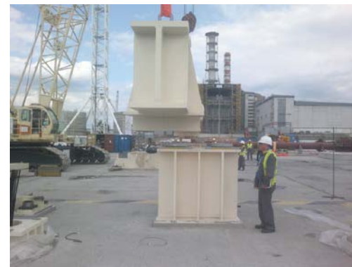
Lifting of Jacking units Set up to the Jacking Tower 3/3
